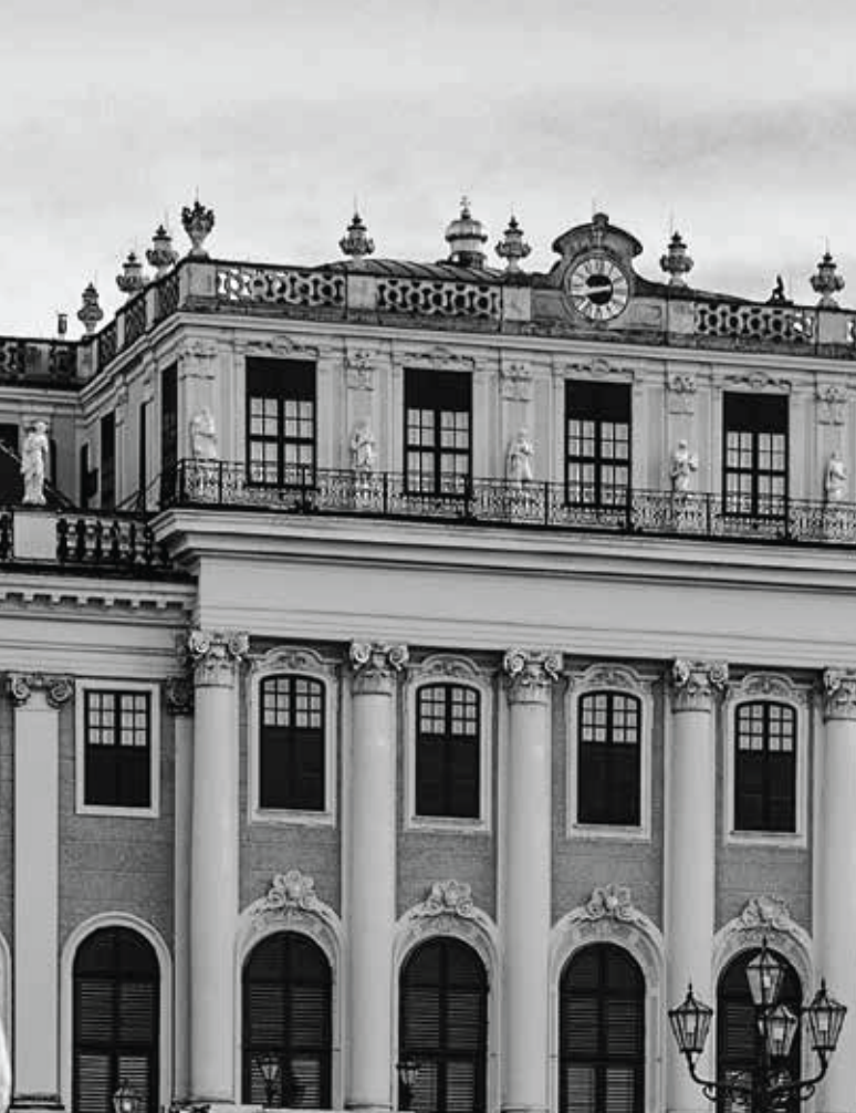
SCHONBRUNN PALACE Boroque architecture
